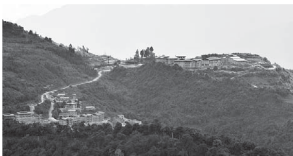
The new ILCS campus in Taktse, Trongsa
